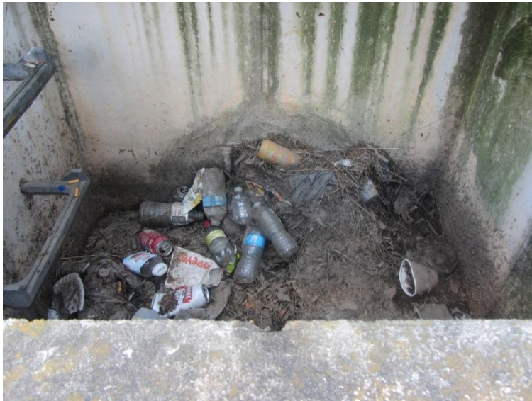
Accumulation of floatables from outfall
