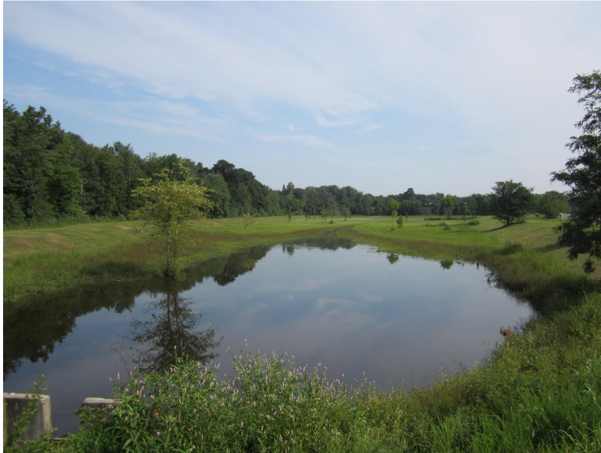
Standing water in detention basin
