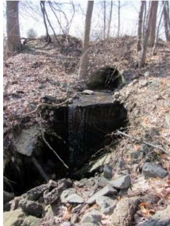
Outlet Destabilization
